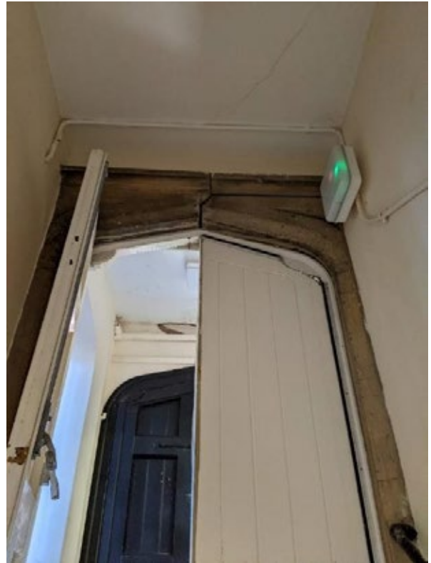
Figure 156: Access door to emergency stairs from unheated space
