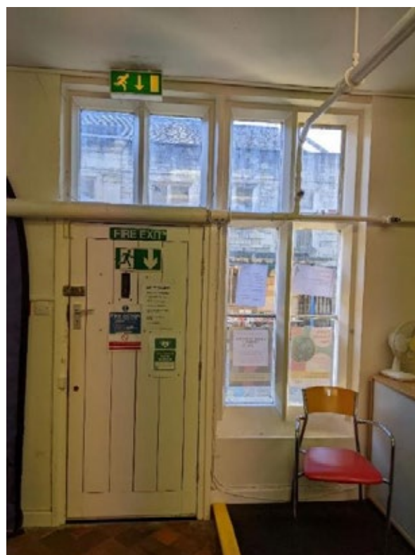
Figure 60: Entrance door at front of building in GF Office 2
