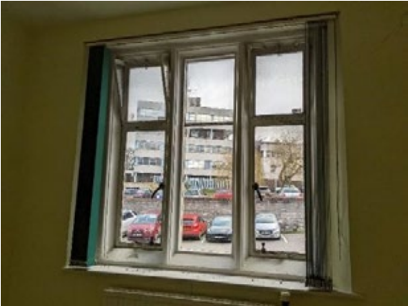
Figure 119: Window in FF Office 5
