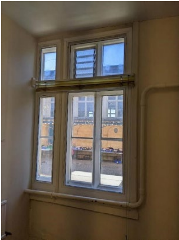
Figure 53: Window in GF Office 1
