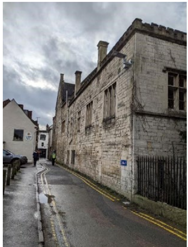
Figure 31: Rear wall, looking down Church Street
