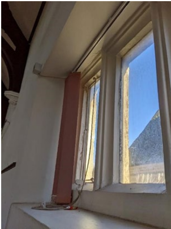
Figure 137: Window in the rear (east) facing wall
