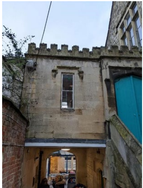
Figure 27: Rear wall of first floor kitchen above walkway
