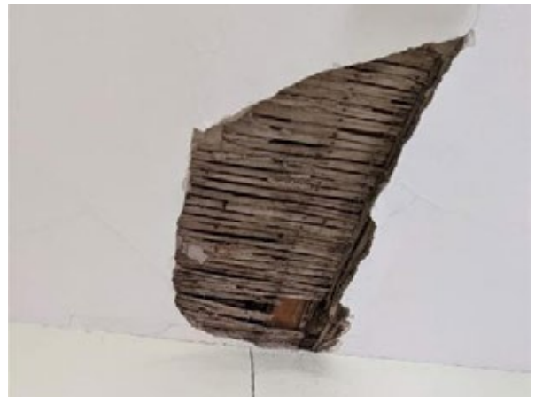
Figure 114: Ceiling in FF Office 4
