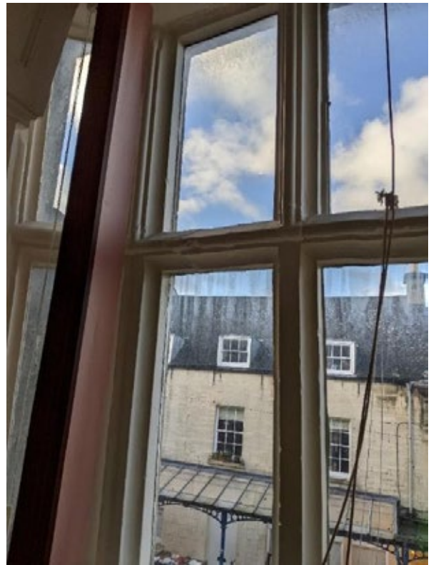
Figure 138: Window in front (west) facing wall
