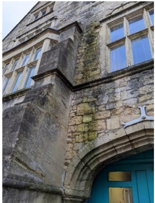
Figure 19: Top of right buttress when facing the building
