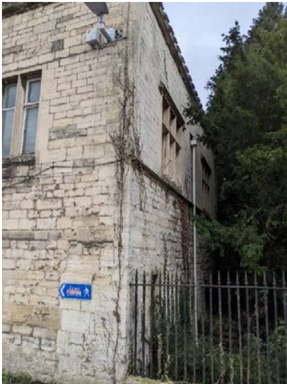
Figure 34: North wall, facing Church
