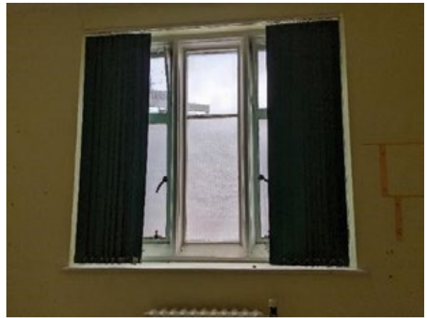
Figure 112: East facing window in FF Office 4 (rear)
