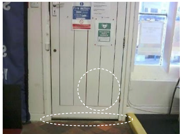
Figure 70: Photograph showing bottom of entrance door into GF Office 2
