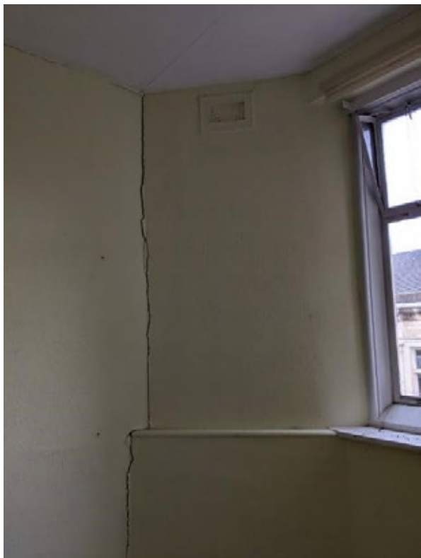
Figure 95: Chimney breast in FF Office 2
