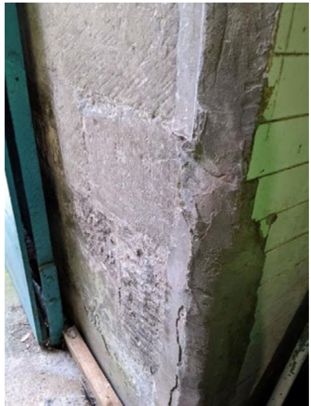
Figure 46: Entrance to Store 3
