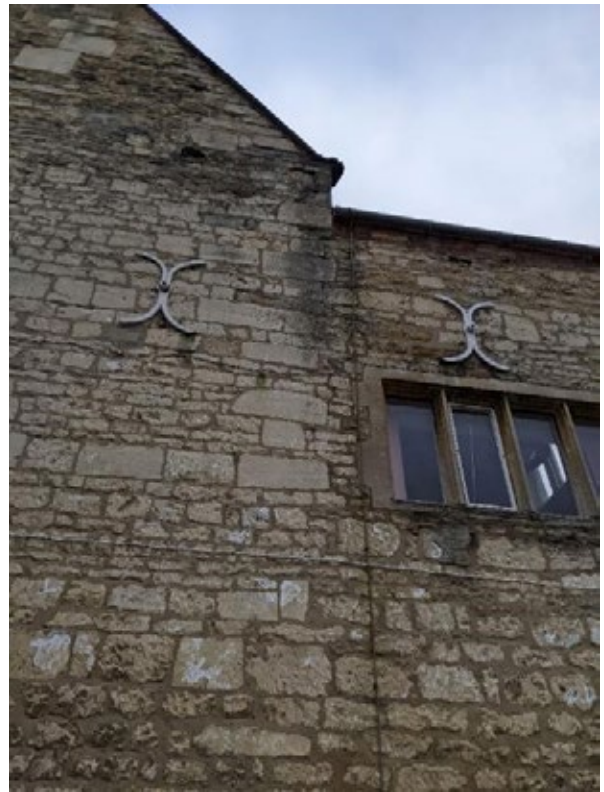
Figure 33: Rear wall of original 16th Century part of building
