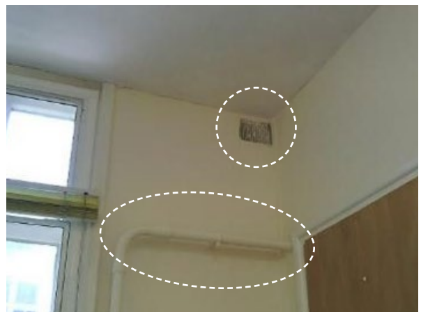
Figure 58: Photograph showing vent and hot water pipe in GF Office 1
