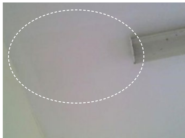
Figure 102: Photograph showing ceiling
