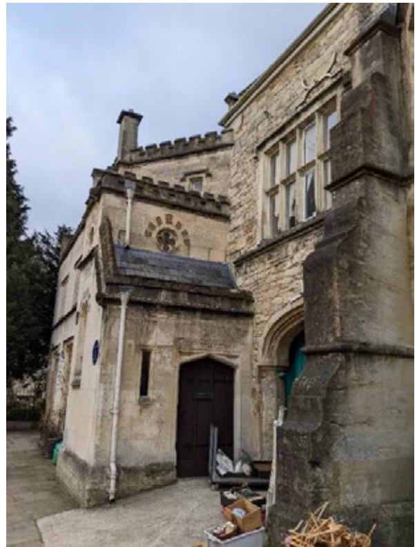
Figure 13: Front view, main entrance door
