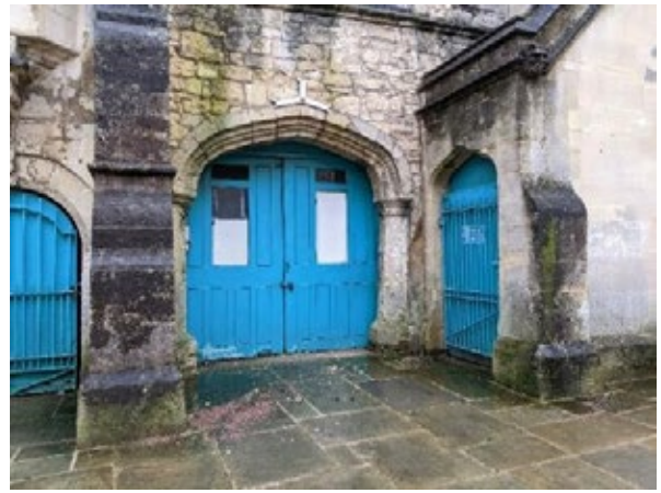
Figure 17: Storage entrances and exit from stairway (far right door)
