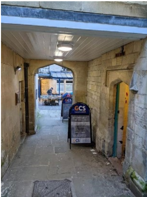
Figure 26: Walkway under first floor kitchen, facing rear of building
