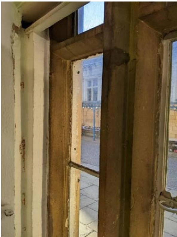
Figure 63: Window frame in GF Office 3
