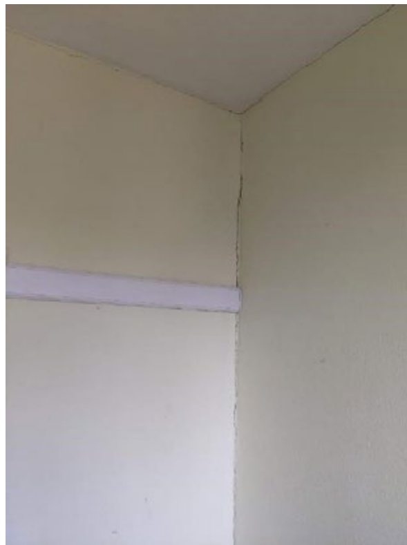
Figure 96: Junction between partition wall to FF Office 1 and corridor
