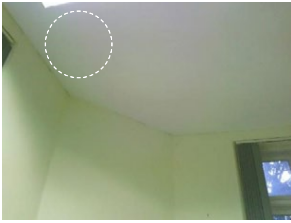
Figure 106: Photograph showing ceiling in FF Office 3
