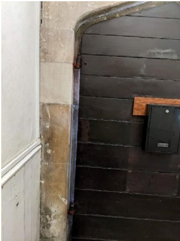
Figure 79: Main entrance door
