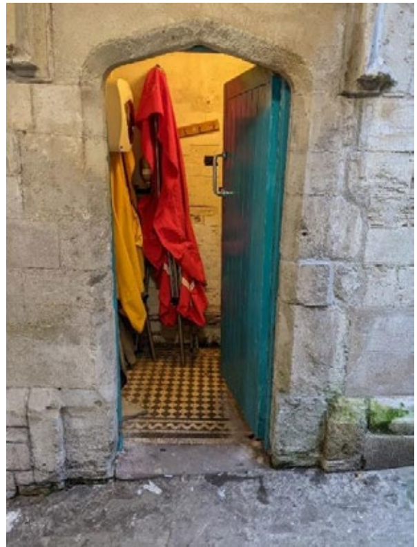
Figure 25: Storage in old outside WC, accessed from walkway under first floor kitchen
