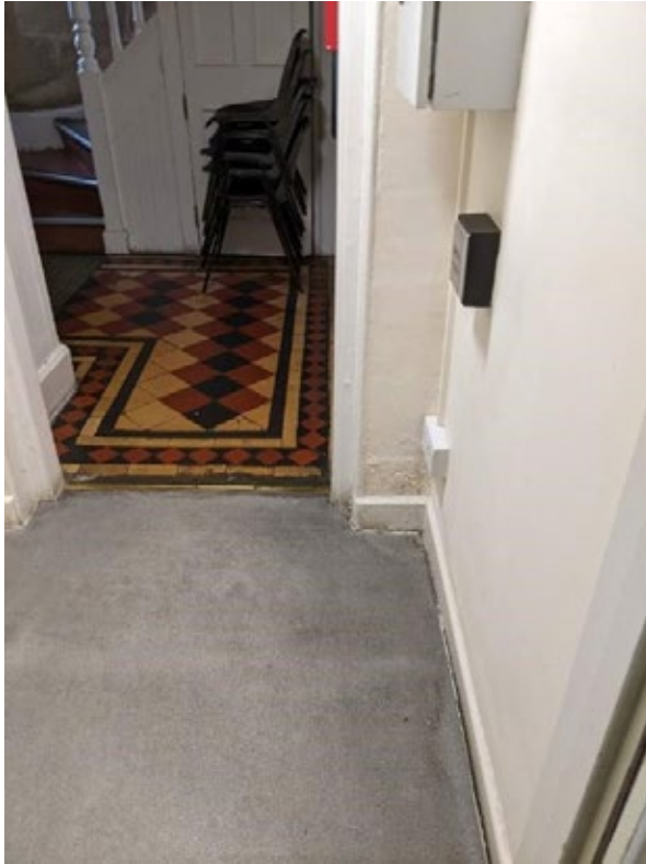
Figure 83: Floor of lobby and access to GF circulation space
