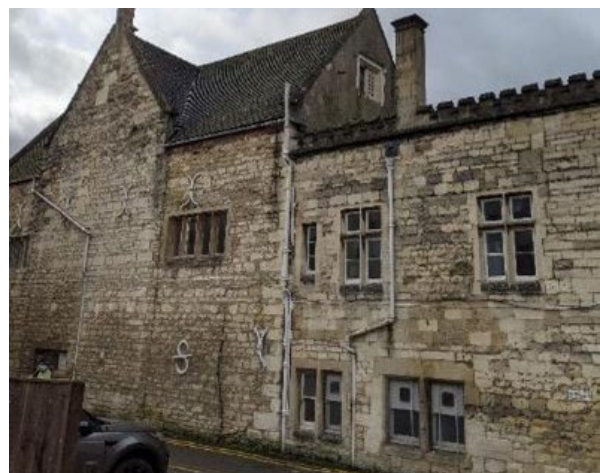
Figure 3: View from Church Street car park (rear)
