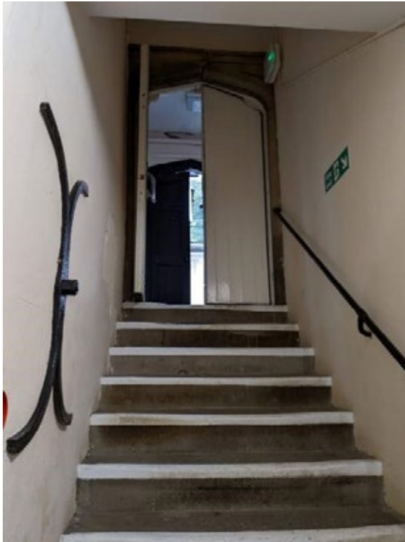
Figure 155: Internal emergency stairs
