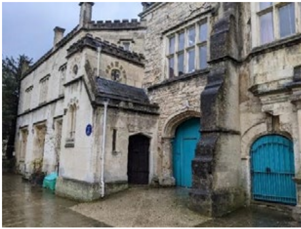
Figure 16: Front entrance and storage entrances
