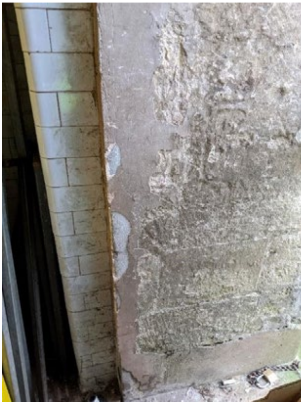
Figure 45: Entrance to Store 3
