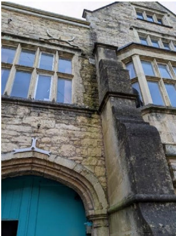
Figure 18: Top of left buttress when facing the building
