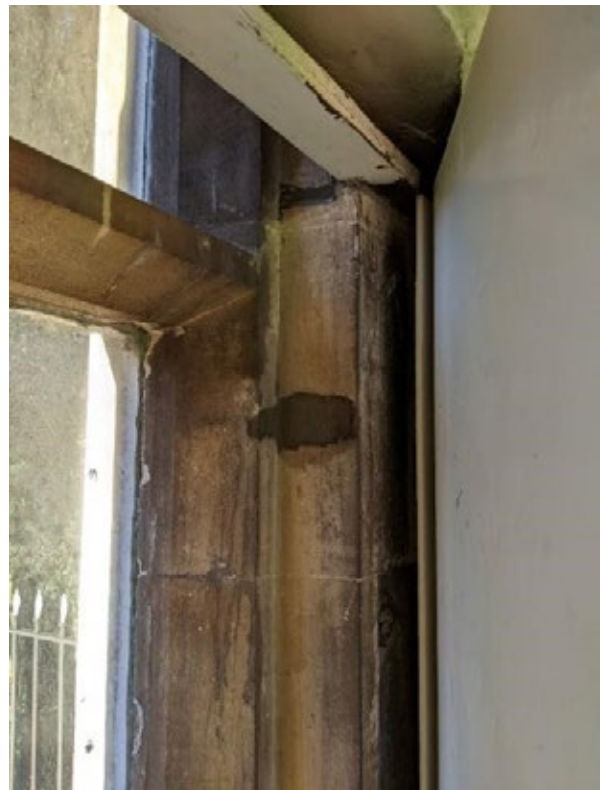
Figure 64: Window frame in GF Office 3
