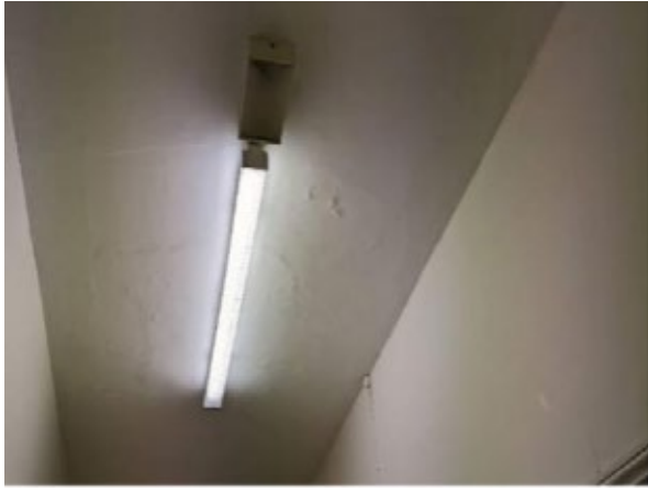
Figure 171: Single 5' T8 light fitting
