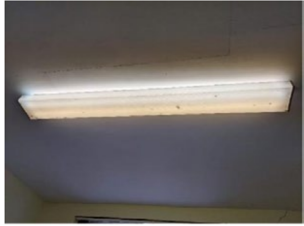
Figure 172: Double 5' T8 light fitting
