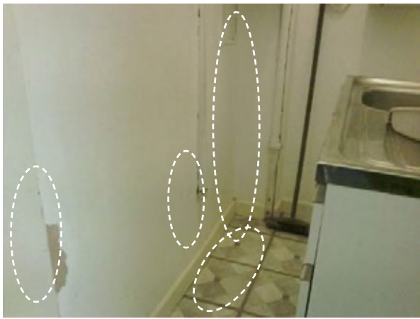
Figure 76: Photograph showing wall and wall junction.
