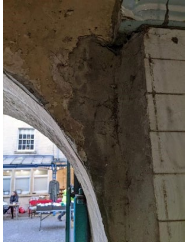
Figure 44: Entrance to Store 3
