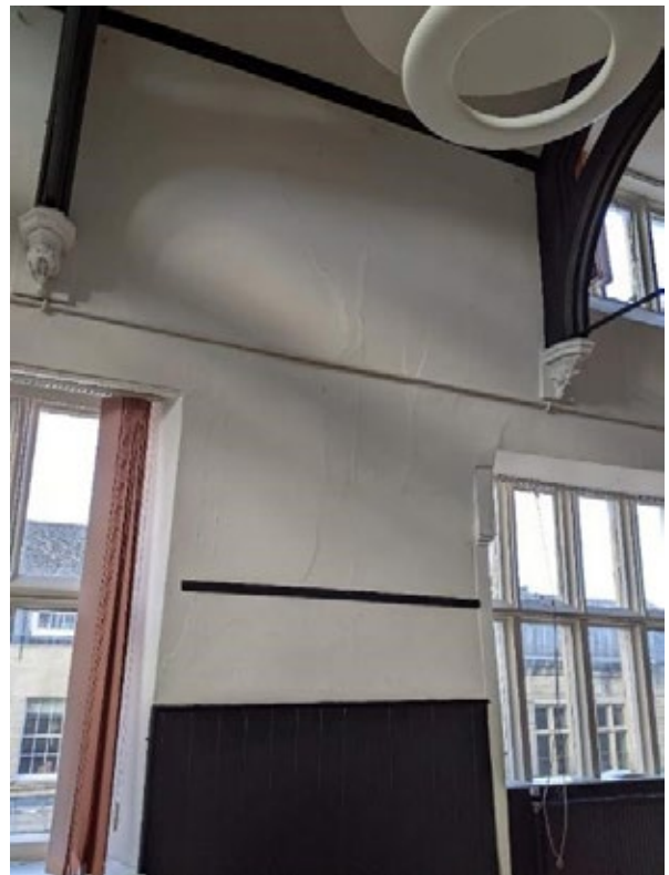
Figure 136: Internal surface of front (west) facing external wall - main facade
