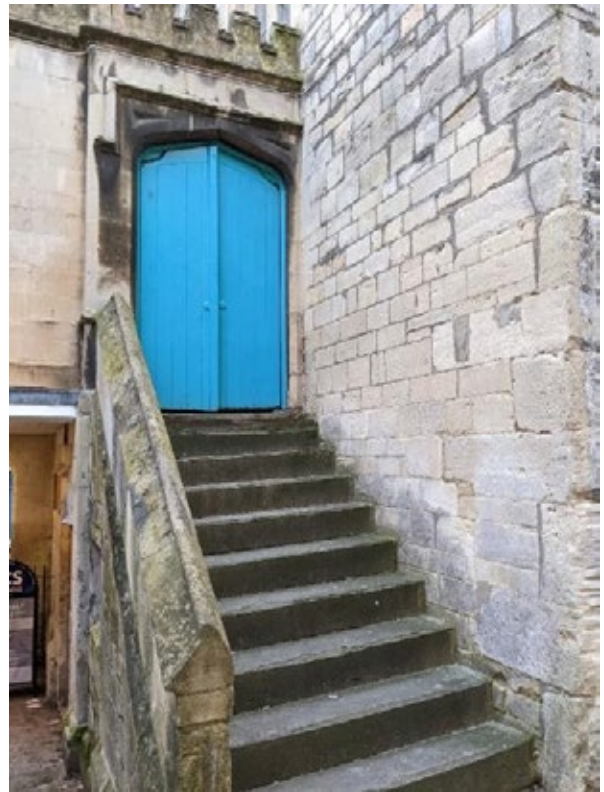
Figure 29: Steps and exist from corridor between first floor meeting room and kitchen
