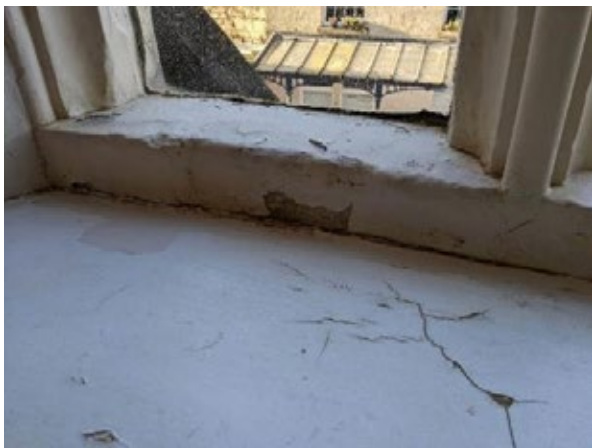
Figure 139: Painted stone window mullion and sill
