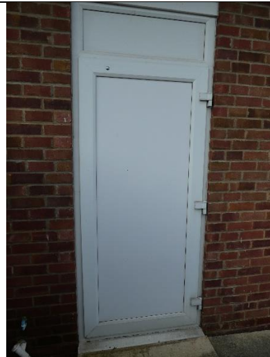
Photo 10 Exit door signage
